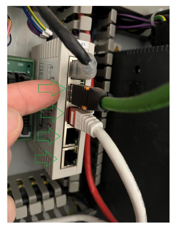
4. Try to switch the ethernet cables around in the switch, as shown in the picture below.
