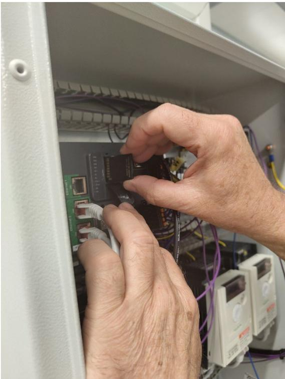
**Step 9.** Wait for 6 LEDs to light up constantly - Then remove the SD card.
