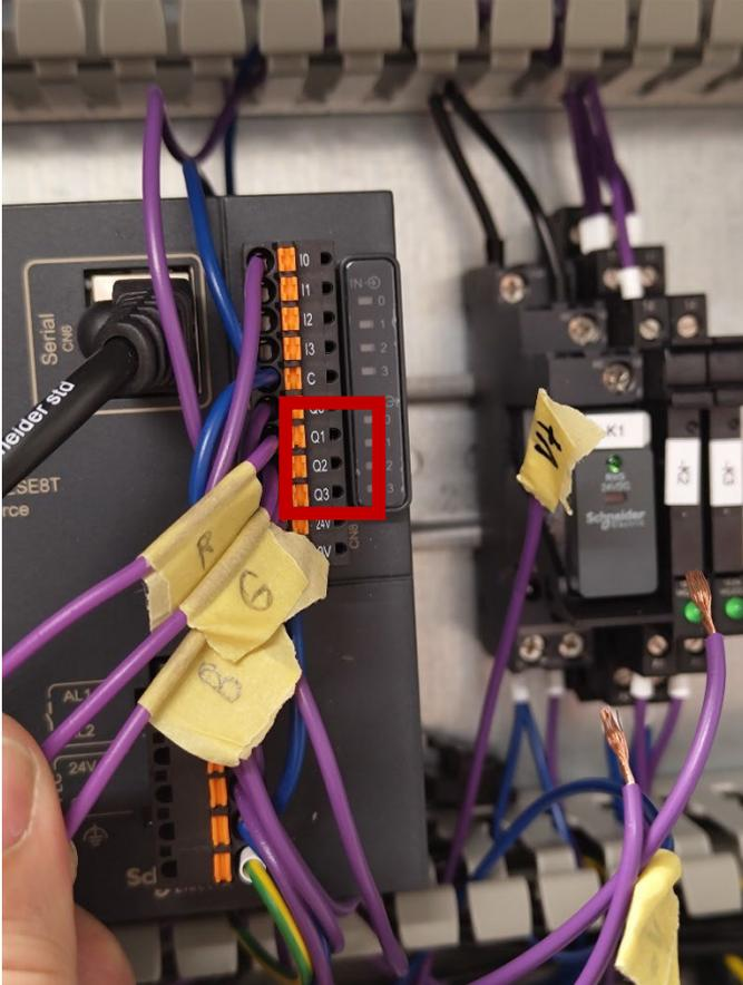
**Step 8.** Insert SD card and switch on white fuse
